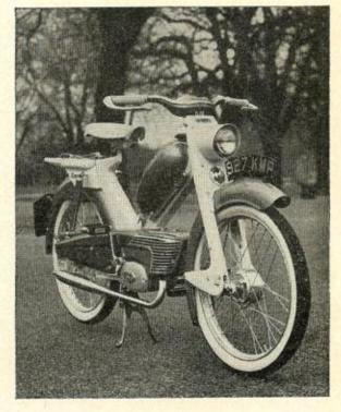
and chain, the pedal drive being independent. The straight tube open frame of heavy gauge tubing has the tank set between the down tubes. Front forks are *Webb* springers. Cycle brakes are used and the lighting equipment and number plates are included in the very down-to-earth price of under £50. (tax included).
