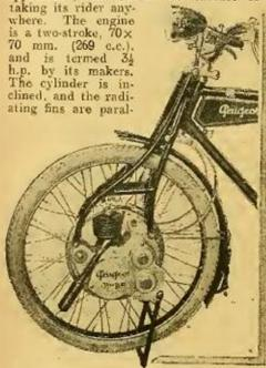
As at the Paris Salon, the front wheel driven Peugeot bicycle attracted much interest at Olympia. The hub is supported on three small pinions, one of which transmits the power.
