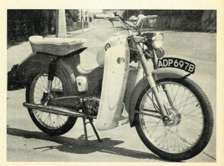
Eighteen inch plated steel rims with 2.25-inch tyres are mounted on light alloy hubs incorporating the hand-operated front and back pedal operated rear brakes.
