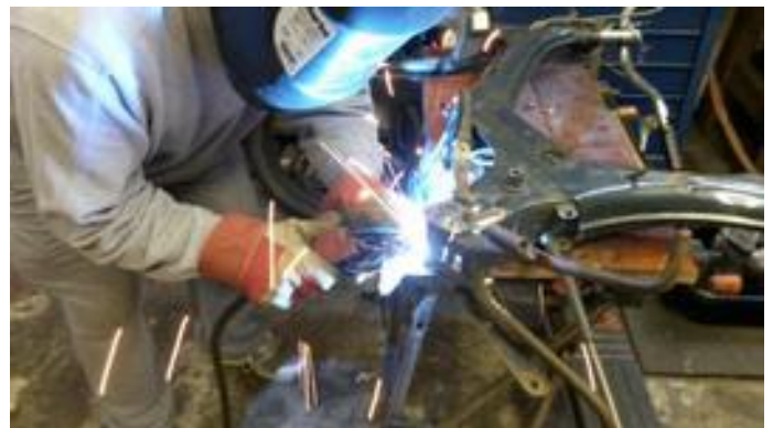
Ken at work on the PC50 frame.
