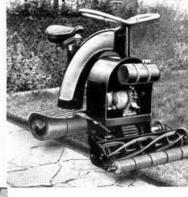
AWNRIDER CUTS MORE VENLY The fully-floating cutter-box naintains a constant cutting height. Vith a pedestrian mower, varying ressure on the guide handles inevitbly causes uneven cutting.
