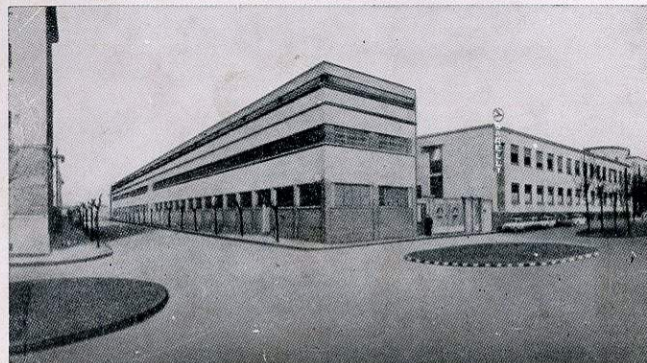
STABILIMENTO MOTORI E.TS MOTEURS ENGINEERING WORKS
