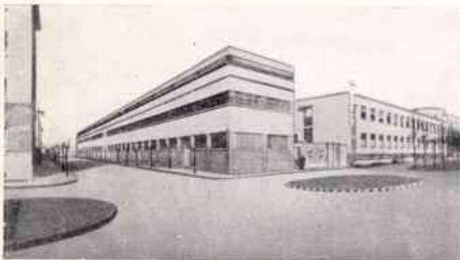
STABILIMENTO MOTORI USINE MOTEURS ENGINEERING WORKS
