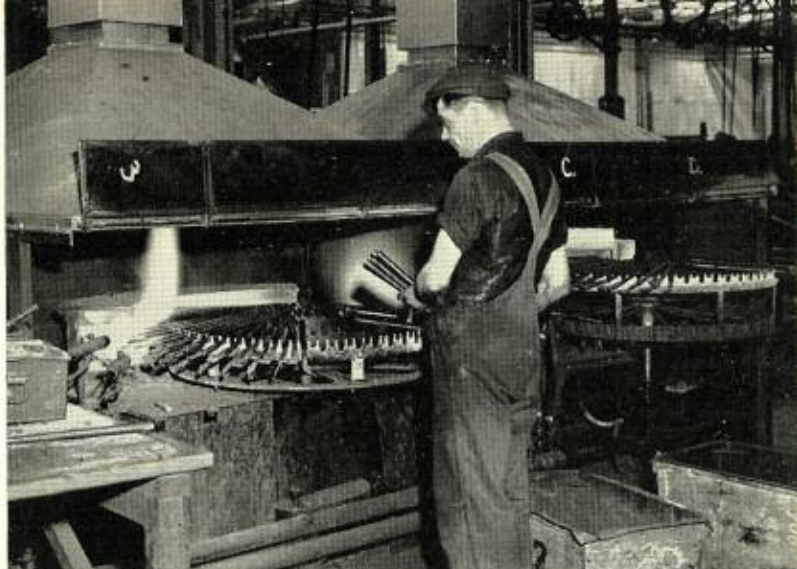
Automatic hearths are used in the stay brazing department
