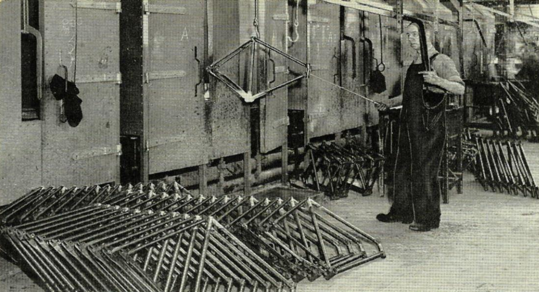
Another view of Raleigh factory, showing how frames are fed into the brazing ovens
