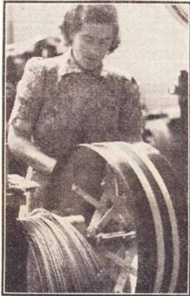
Hand building the Safety Speed tyre
