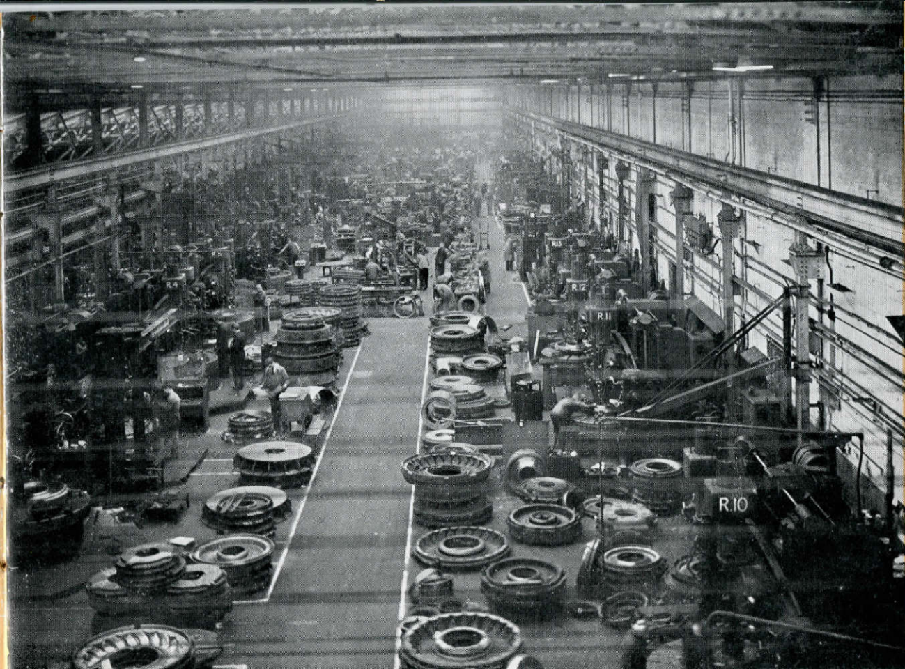
One of the Machine Shop Bays
