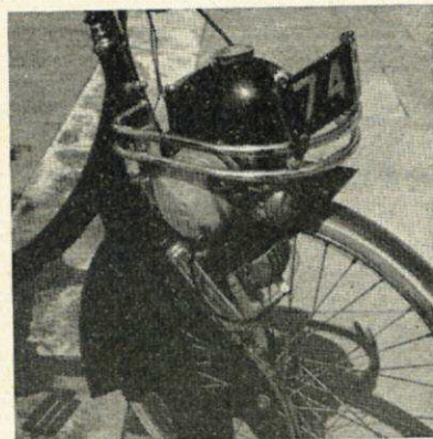
LEFT: A real stand, a sturdy carrier, built-in lock and enclosed chain drive are good features. RIGHT: The power unit is neat, light and well guarded.
